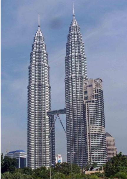
Fig. 17 – Petronas Towers, Kuala Lumpur, 1996
