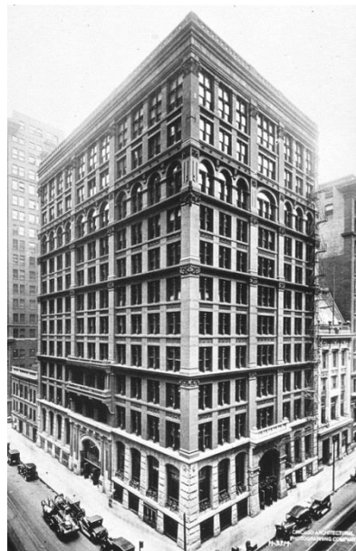
Fig. 2 - Home Insurance Building, Chicago, 1884
