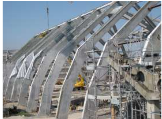
Figure 20 - Reinforcement of Corpo C columns
