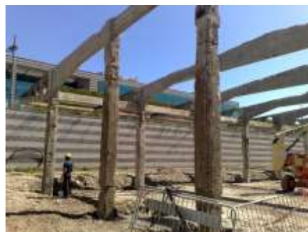
Figure 7 - Corpo C - Original reinforcements
