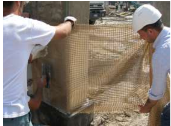
Figure 18 – Shear reinforcement of Corpo B base
