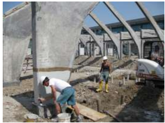
Figure 19 – Shear reinforcement of Corpo B base
