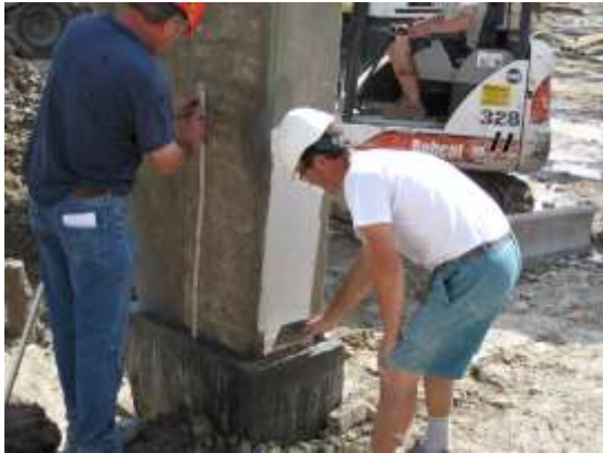
Figure 18 – Shear reinforcement of Corpo B base
