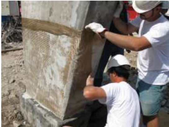
Figure 19 – Shear reinforcement of Corpo B base
