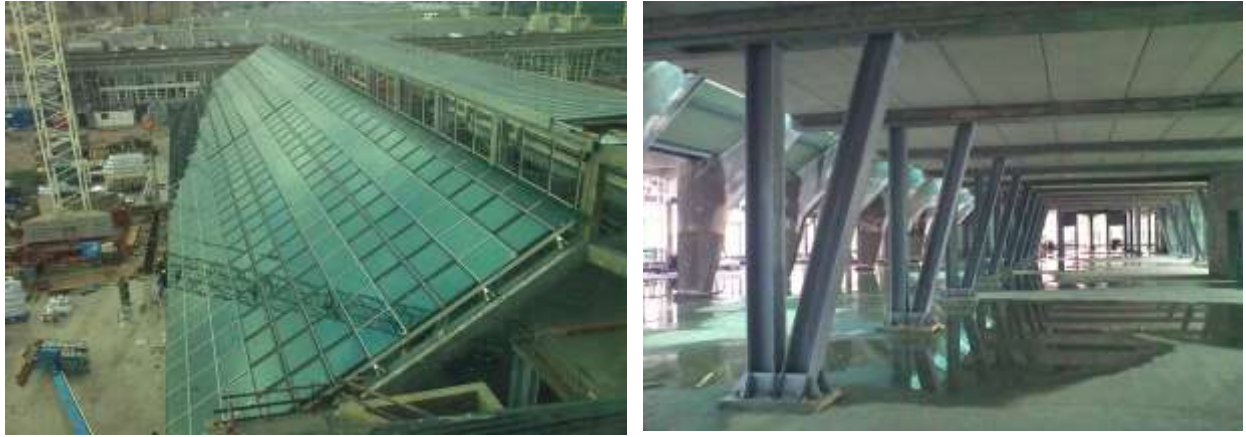
Figure 24 - Corpo B – facades and new columns
