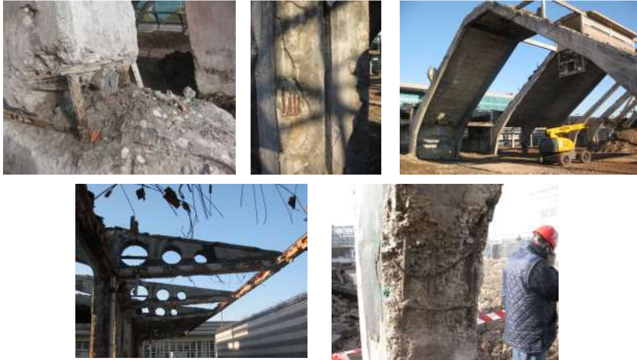
Figure 6 - Building before retrofitting
