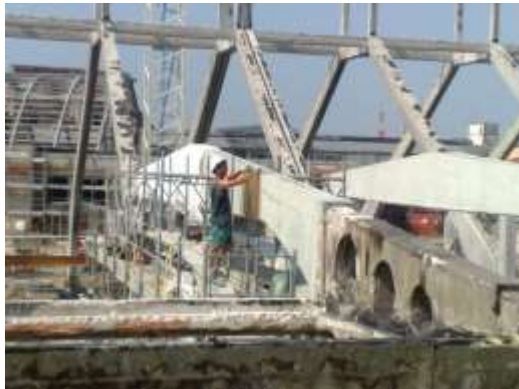
Figure 20 - Reinforcement of Corpo C columns
