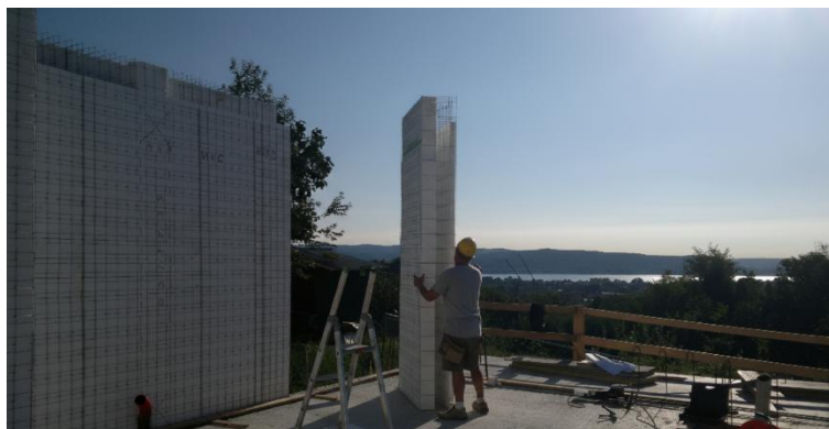
Posa in opera
