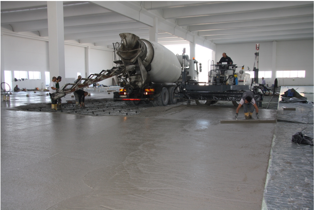
Posa in opera mediante laser screed.
