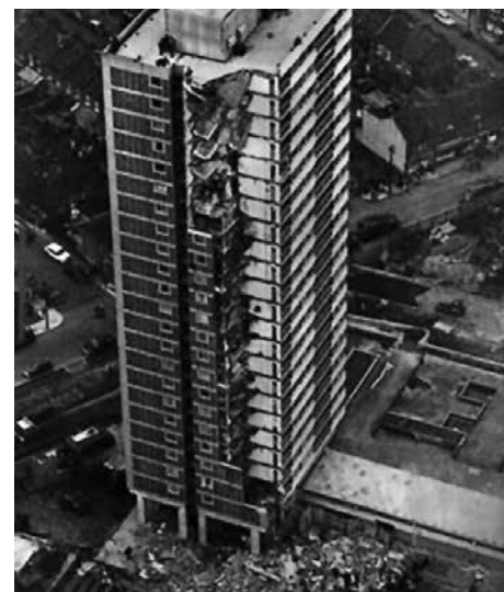
Figura 1 – Collasso Roman Point ( http://www.failedarchitecture.com/the-down-fall-of-british-modernist-architecture/ )
