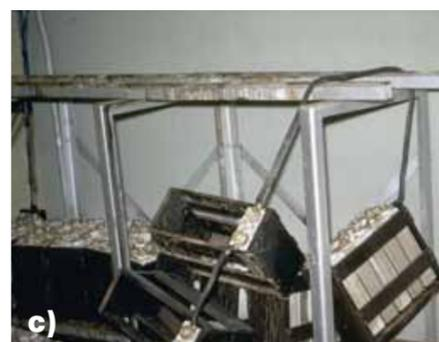
Figure 1 – Examples of earthquake damages; a) A sheared pipe, b) A broken sprinkler head, c) Collapsed emergency battery racks
