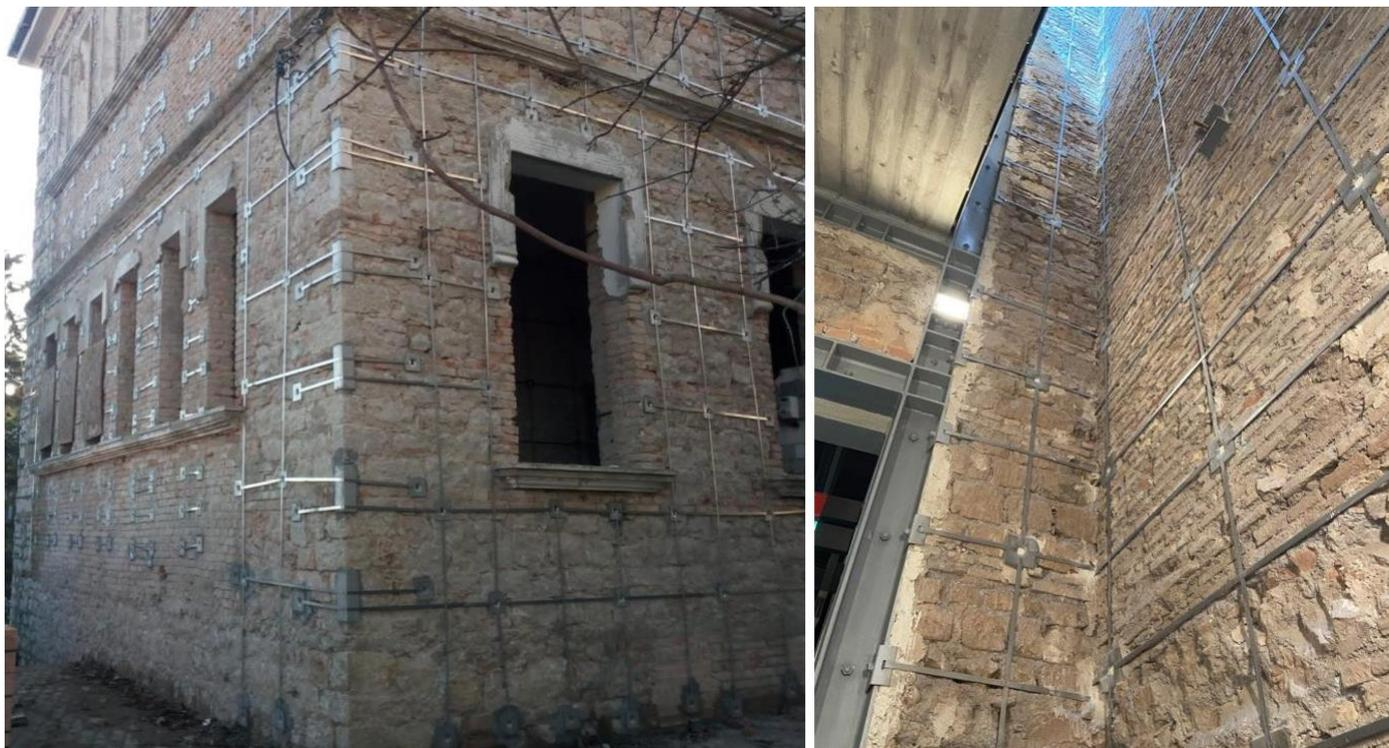
FIGURA 6: LA MAGLIA CAM<sup>®</sup> IN CORRISPONDENZA DEGLI INCROCI MURARI REALIZZA IL VINCOLO NEI CINEMATISMI DI RIBALTAMENTO
