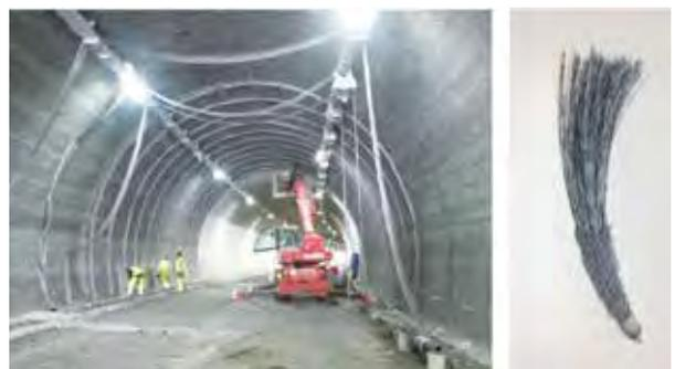
Fig. 5. Systematic lining reinforcement by Steel Net G220 and detailing of connector SFIX G 12
