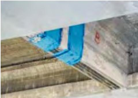
Fig. 6. Strengthening of the transversal RC beams.
