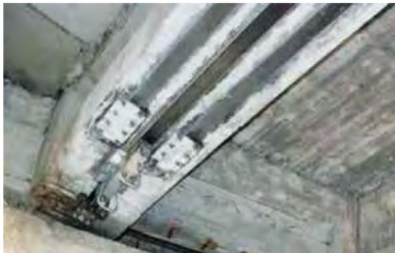
Fig. 9. Removal of the hydraulic jack and provisional anchorages 48 hours after the prestressing process.
