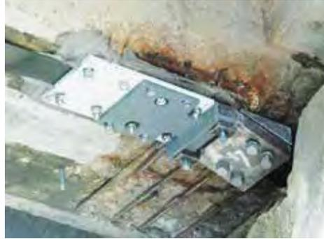
Fig. 7. Insertion of the laminate into the steel anchorage at the fixed end.
