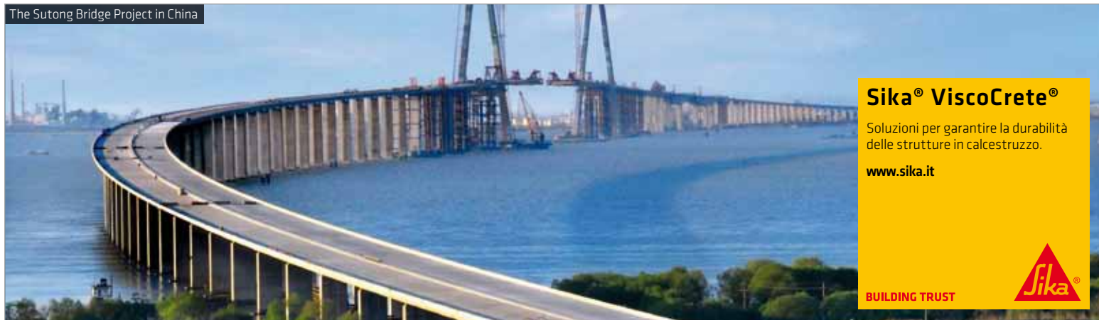
The Sutong Bridge Project in China
